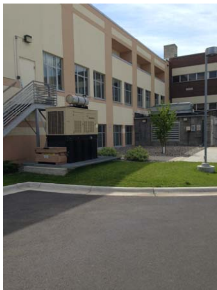
Examples of generators/equipment that are not enclosed
